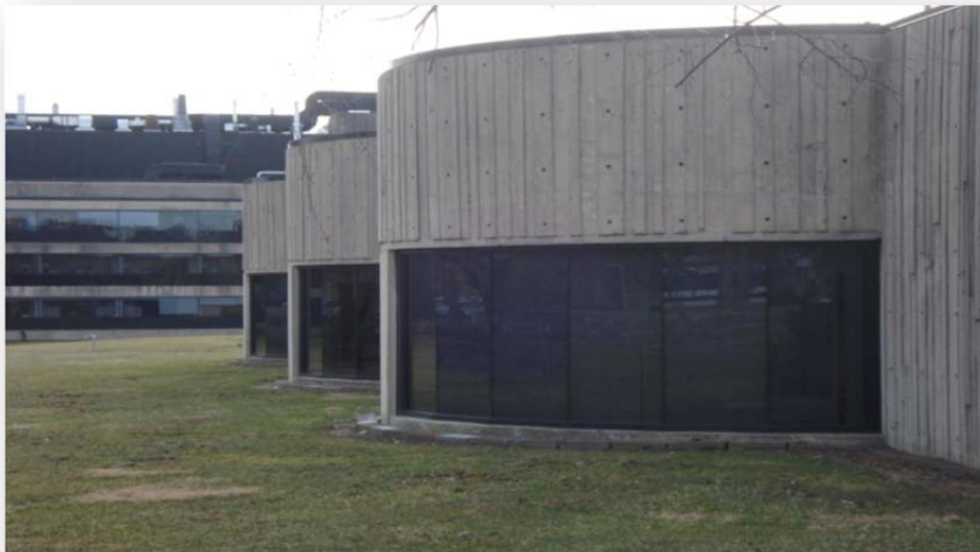
Digitech's Colocation is in a Tier 3 Data Center built to withstand a nuclear attack
